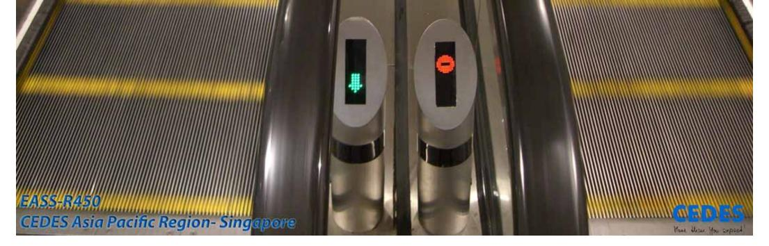
CEDES presence sensor is operated with invisible infrared light. If there is an object in the field of view of the sensor, part of the light from the emitter is scattered back to the receiver. The Cedes presence sensor is house in a stainless steel housing which will be used to detect the presence of person, trolleys in front of the Escalator or Auto walk.
